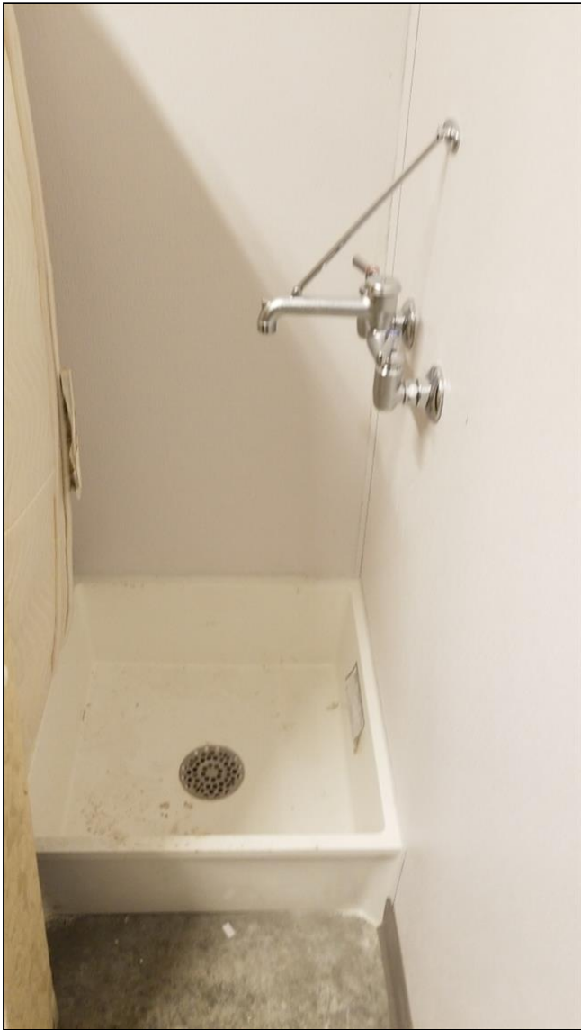
3.0 Item 6(Picture) 1st floor, larger
