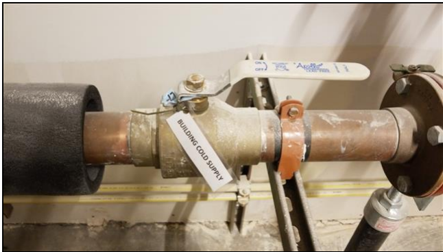
5.3 Item 1(Picture) 1st floor utility room.
